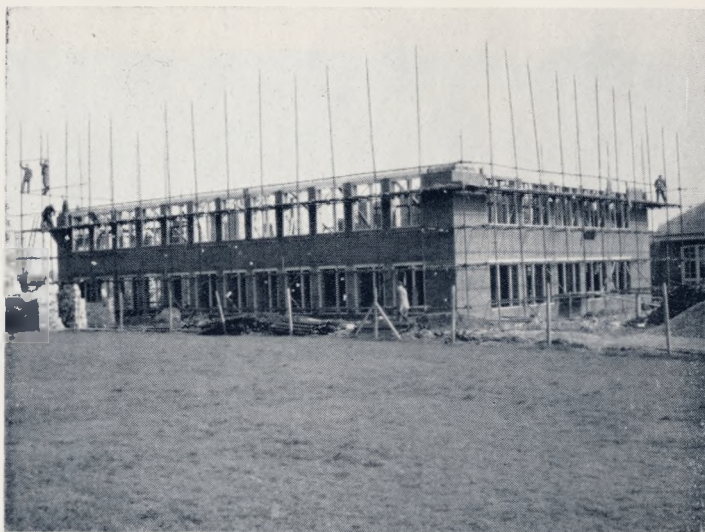
PROGRESS ON THE NEW SCIENCE BLOCK
